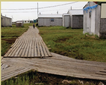
Wooden boardwalks connect houses and community buildings in Newtok, Alaska, and keep residents from sinking into the muddy ground as they walk or ride around the village.
